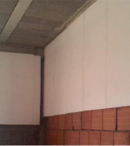
Figure 30.- Placement des plaques de l'EPS. (Source: ADEREE)
